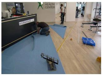
This is a typical example of installing a PVC floor coverings onto an underlay using UZIN KE 2000 S.
