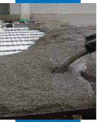
Pouring concrete with the addition of Mapefibre NS12 to counter plastic shrinkage
