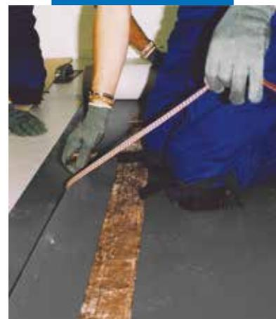
Removal of the cutted portion of Mapelay
