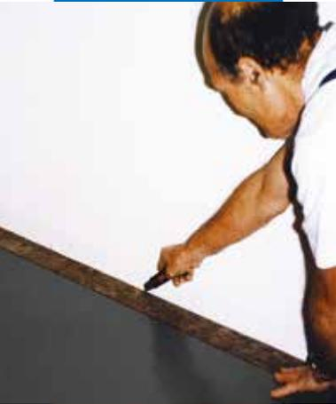
Laying Mapelay and formation of a 5-10 mm joint in correspondence with the constraints of the floor
