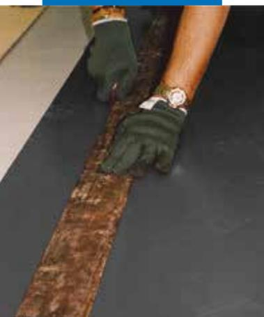
Cutting the joint between sheets of Mapelay
