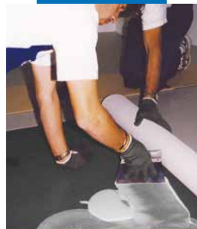
Laying rubber floor covering on Mapelay sheets using Adesilex G19. N.B. The joints between the sheets of rubber floorings are staggered with respect to the joints in the sheets of Mapelay
